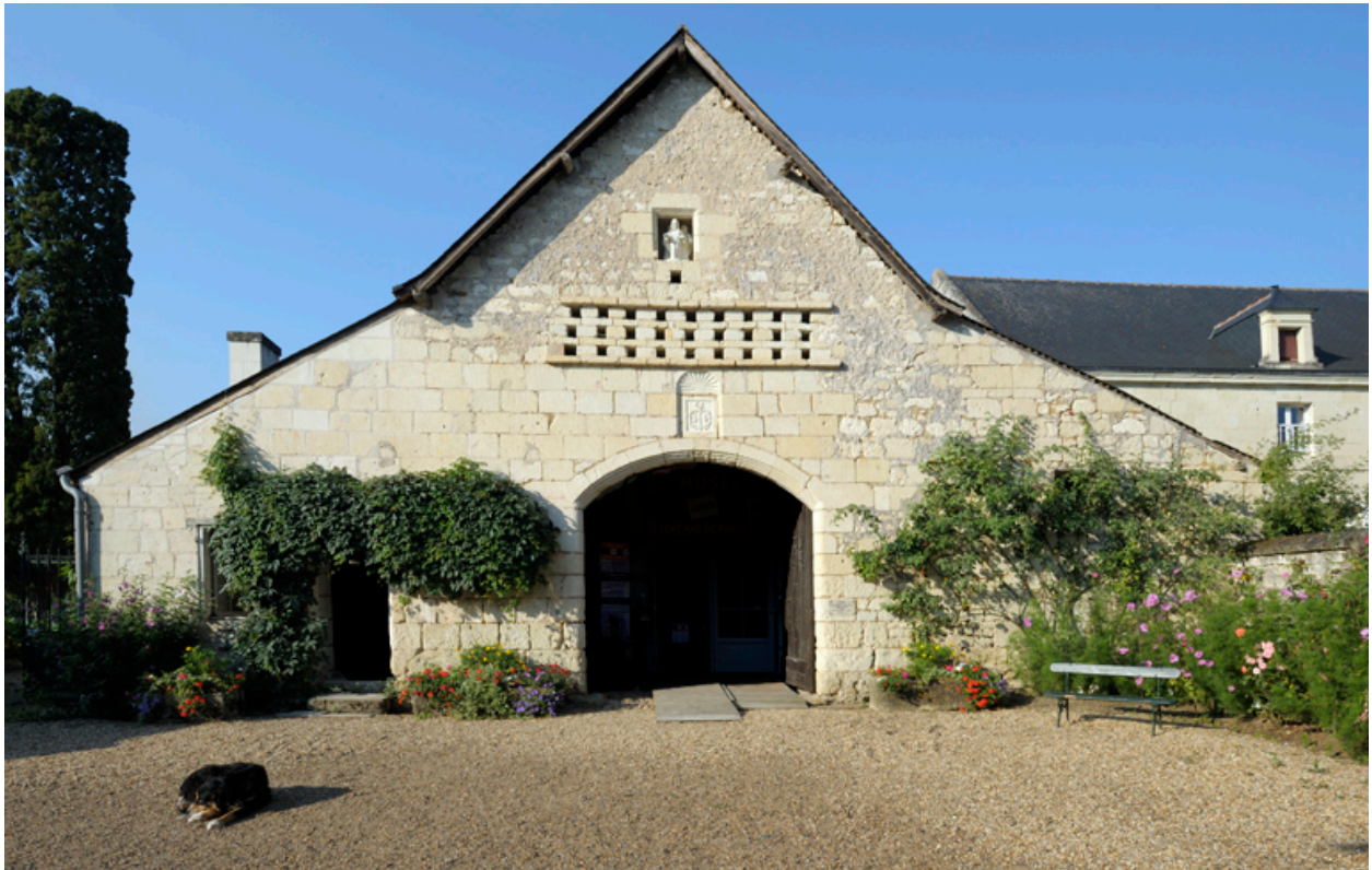
Grange, façade principale.
