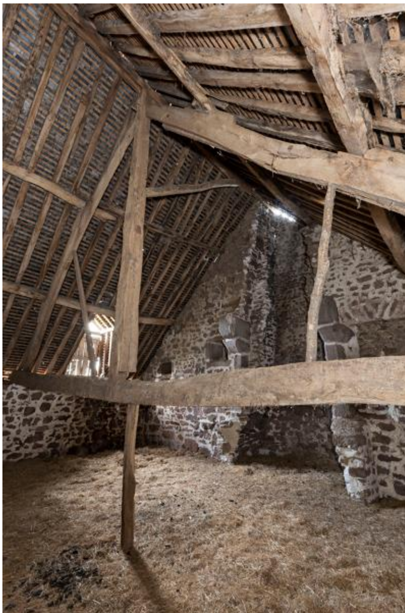
Logis central, manoir originel, charpente.
