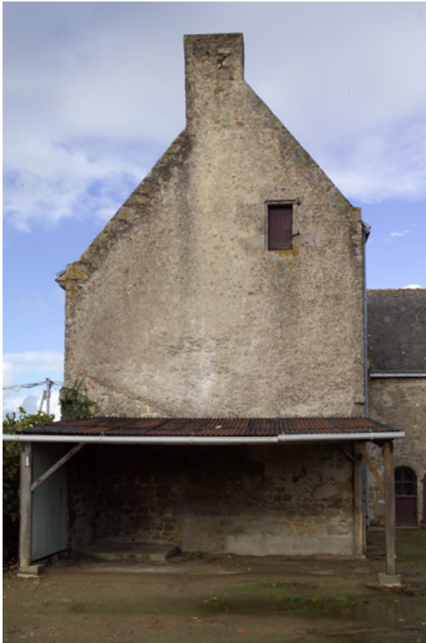
Aile sud, pignon oriental.
