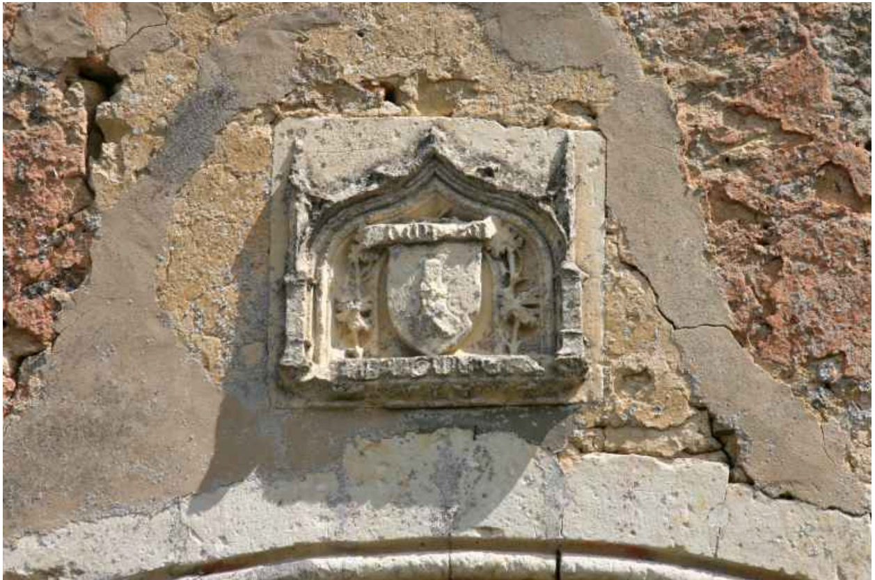
Façade occidentale : armoiries.
