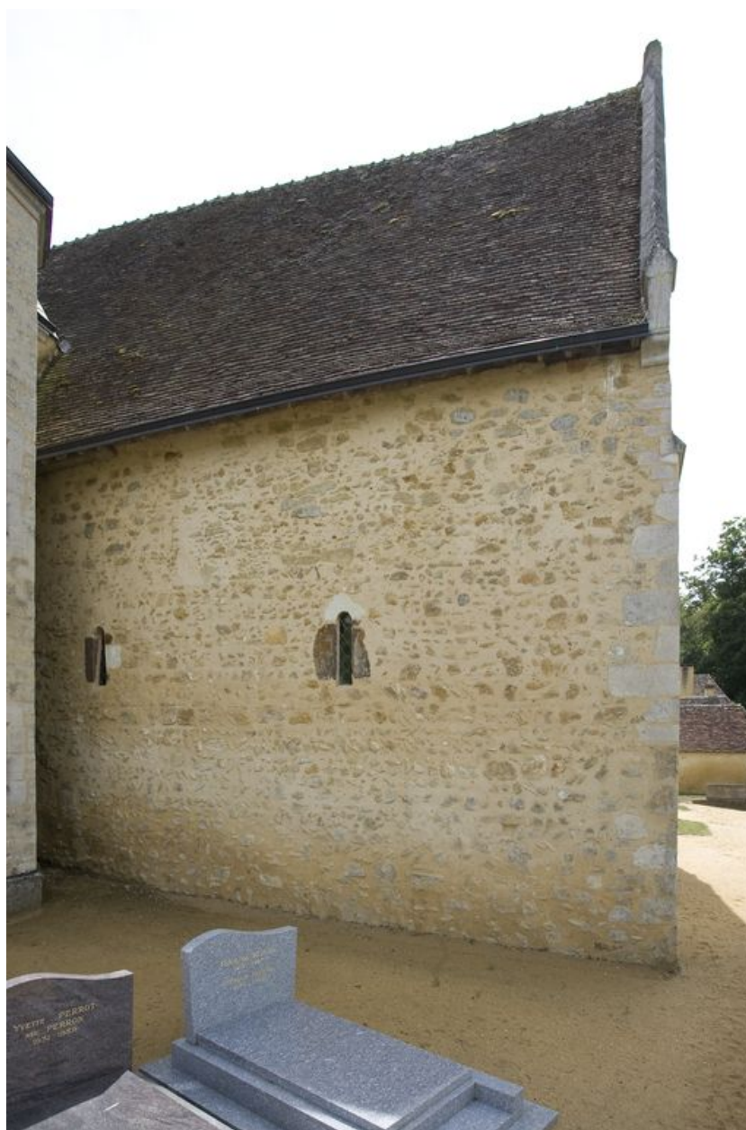
Nef, élévation nord, XIe siècle.
