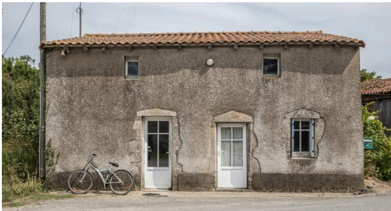
Habitation double. La Pichaudière, Saint-Hilaire-de-Clisson. Cadastre 2018, ZR 01-133.
