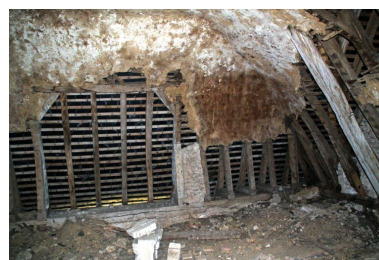
Comble. Phot. Jean-Baptiste Darrasse IVR52_20107200420NUCA
