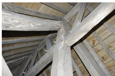
Logis. Charpente. Phot. Denis Pillet IVR52_20094401268NUCA
