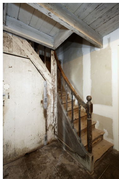
Logis. Escalier. Phot. Denis Pillet IVR52_20094401252NUCA
