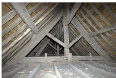
Logis. Charpente. Phot. Denis Pillet IVR52_20094401266NUCA
