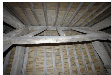
Logis. Charpente. Phot. Denis Pillet IVR52_20094401267NUCA
