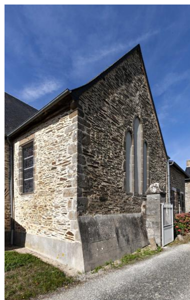
Transept, bras sud. Phot. Yves Guillotin IVR52_20205300241NUCA
