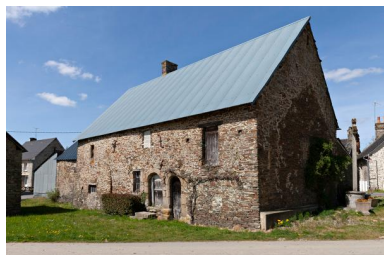
10 Montoger (2023 ZC 86), logis-étale Phot. Yves Guillotin IVR52_20195300446NUCA
