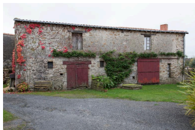
Habitation double, AW01-733, cadastre 2018. Phot. Denis Pillet IVR52_20154400673NUCA
