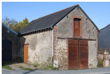
Magasin. Phot. Armelle Maugin IVR52_20254900241NUCA
