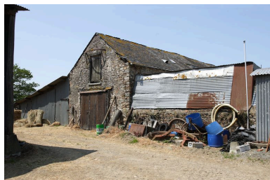
La remise. Phot. François Lasa IVR52_20055301714NUCA
