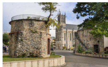
Les chenils. Phot. Pierre-Bernard Fourny IVR52_20215301157NUCA
