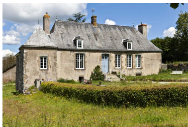
Façade sud. Phot. Yves Guillotin IVR52_20215300626NUCA
