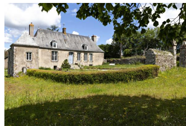
Façade sud. Phot. Yves Guillotin IVR52_20215300625NUCA
