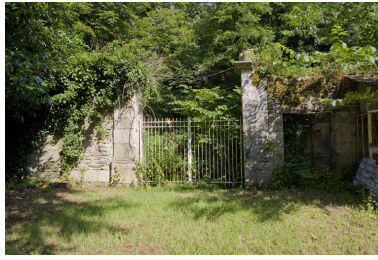
Jardin. Portail. Phot. Denis Pillet IVR52_20084402181NUCA
