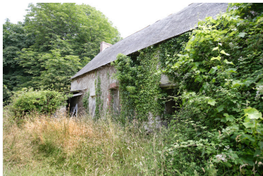
Communs. Façade est. Phot. Denis Pillet IVR52_20084402206NUCA
