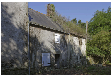
Aile sud. Façade ouest. Phot. Denis Pillet IVR52_20084402167NUCA
