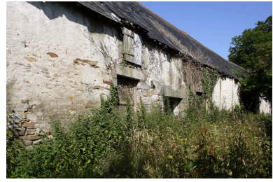
Communs. Façade ouest. Phot. Denis Pillet IVR52_20084402188NUCA
