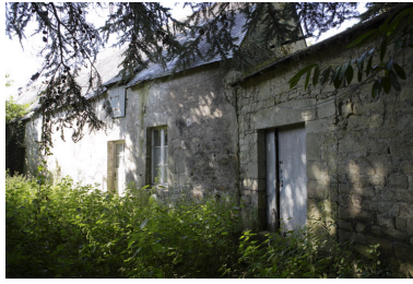
Communs. Façade ouest. Phot. Denis Pillet IVR52_20084402187NUCA
