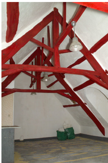
Comble, portion orientale. Phot. Denis Pillet IVR52_20054402364NUCA
