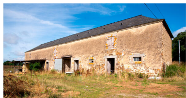
La ferme. Phot. Pierre-Bernard Fourny IVR52_20235300983NUCA
