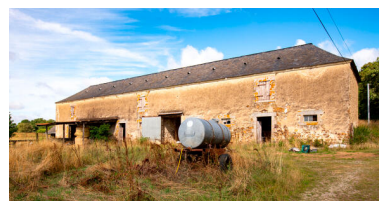
La ferme. Phot. Pierre-Bernard Fourny IVR52_20235300982NUCA
