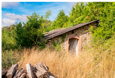
La serre. Phot. Pierre-Bernard Fourny IVR52_20235300967NUCA
