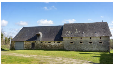
La grange-étable. Phot. Pierre-Bernard Fourny IVR52_20225300287NUCA
