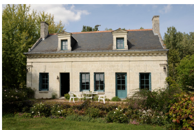
Façade principale. Phot. Bruno Rousseau IVR52_20114902424NUCA
