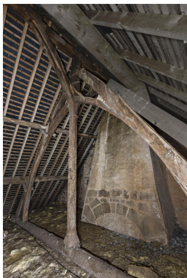
Charpente. Phot. Yves Guillotin IVR52_20195301265NUCA
