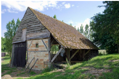
Hangar. Phot. Yves Guillotin IVR52_20107202408NUCA
