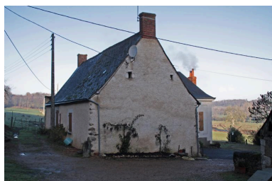
Maison, pignon est. Phot. Jean-Baptiste Darrasse IVR52_20097201667NUCA
