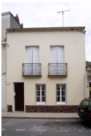
La façade antérieure. Phot. Denis Pillet IVR52_20034400557NUCA
