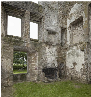
Corps de logis sud. Phot. Yves Guillotin IVR52_20215301393NUCA
