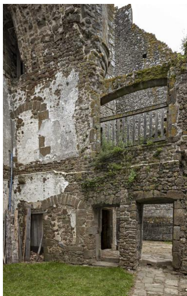
Corps de logis sud. Phot. Yves Guillotin IVR52_20215301395NUCA
