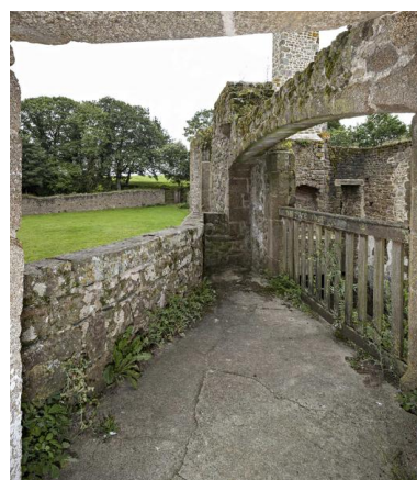
Courtine ouest. Phot. Yves Guillotin IVR52_20215301396NUCA
