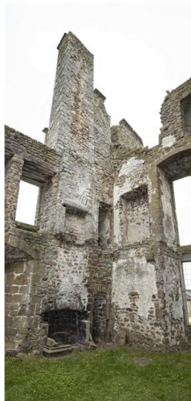
Corps de logis sud. Phot. Yves Guillotin IVR52_20215301394NUCA
