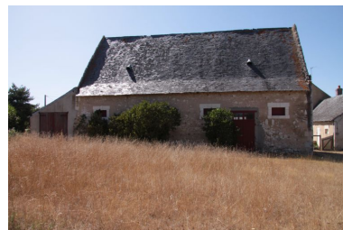
La grange, mur est. Phot. Jean-Baptiste Darrasse IVR52_20097200462NUCA
