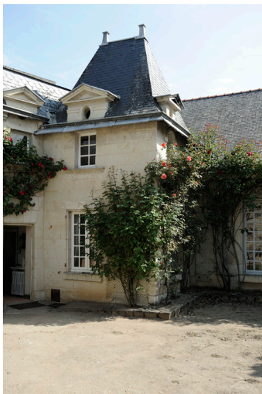
Pavillon d'angle. Phot. Bruno Rousseau, Phot. Youenn Communeau IVR52_20114901683NUCA
