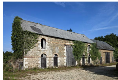
Etable-grange ouest. Phot. Yves Guillotin IVR52_20215301492NUCA
