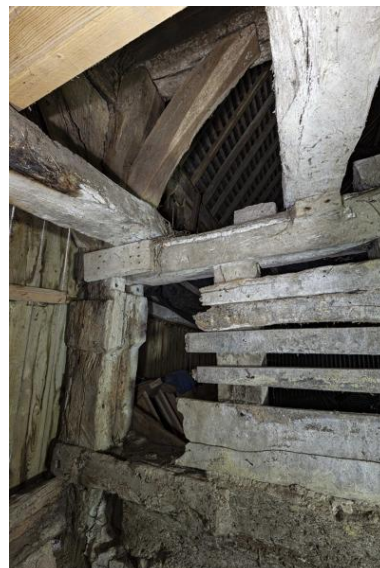
Cloison de refend de la grange. Phot. Yves Guillotin IVR52_20205300407NUCA
