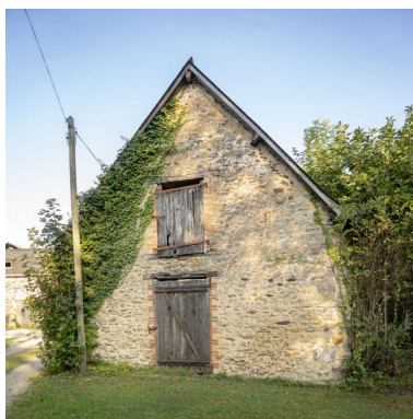
La grange. Phot. Pierre-Bernard Fourny IVR52_20215301220NUCA
