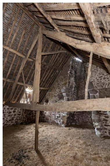
Logis central, manoir original, charpente. Phot. Yves Guillotin IVR52_20195300560NUCA
