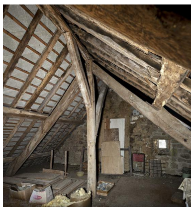
Logis sud, charpente. Phot. Yves Guillotin IVR52_20215301766NUCA
