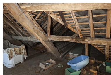
Logis sud, charpente. Phot. Yves Guillotin IVR52_20215301768NUCA
