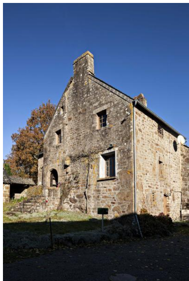
Logis sud, mur-pignon. Phot. Yves Guillotin IVR52_20215301758NUCA
