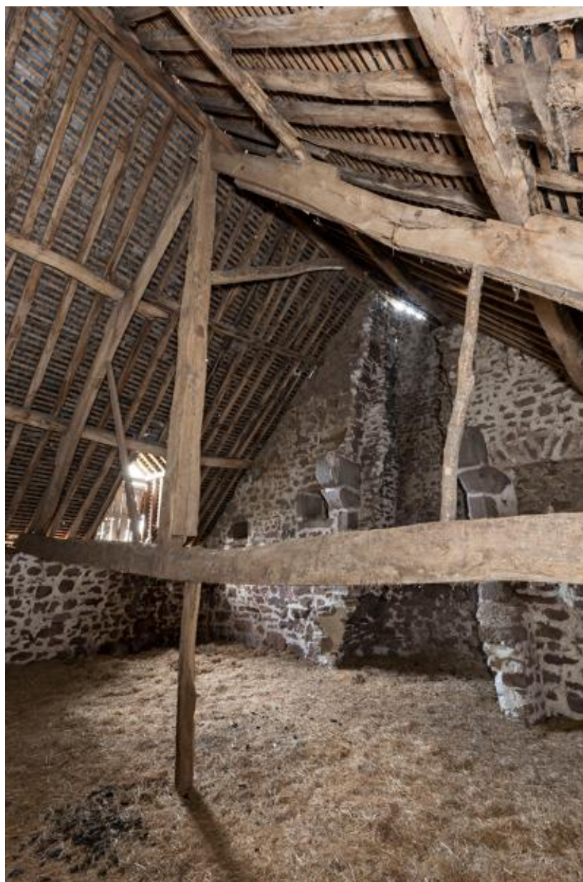
Logis central, manoir originel, charpente.
