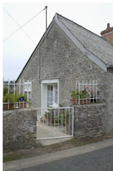
La mur-pignon ouest. Phot. François Lasa IVR52_20045303275NUCA
