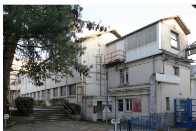
Atelier de fabrication 2. Phot. Denis Pillet IVR52_20094401498NUCA
