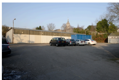
Entrepôt industriel 3. Phot. Denis Pillet IVR52_20094401516NUCA
