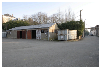
Entrepôt industriel 2. Phot. Denis Pillet IVR52_20094401515NUCA
