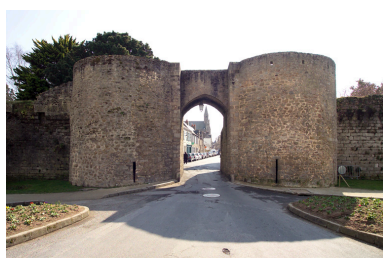
Porte Vannetaise. Phot. Denis Pillet IVR52_20064402096NUCA
