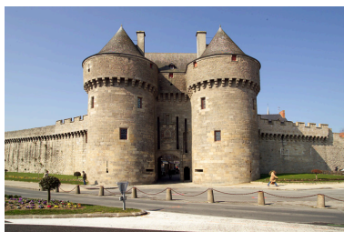
Porte Saint-Michel. Phot. Denis Pillet IVR52_20064402021NUCA
