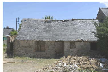
La façade principale. Phot. François Lasa IVR52_20045301945NUCA
