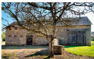
La grange-étable. Phot. Pierre-Bernard Fourny IVR52_20235300297NUCA
