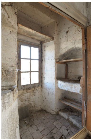
Etage, salle nord. Cabinet nord. Phot. Bruno Rousseau IVR52_20124901517NUCA
