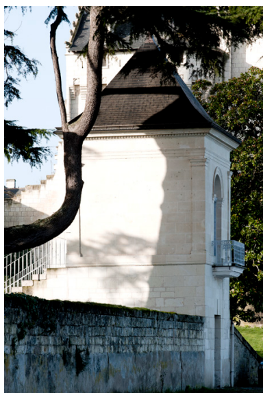
Pavillon : face est. Phot. Bruno Rousseau IVR52_20124900052NUCA
