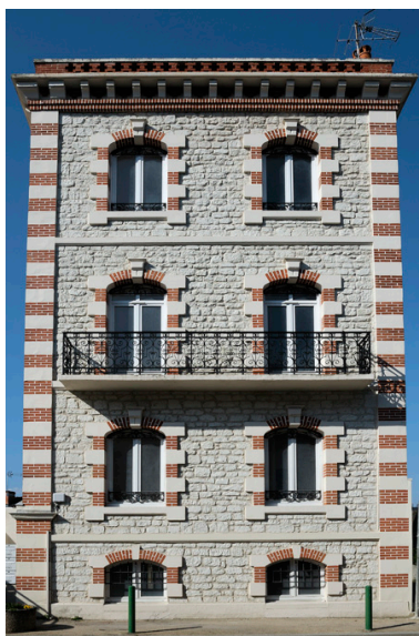
Façade principale Phot. Bruno Rousseau, Phot. Youenn Communeau IVR52_20114900636NUCA
