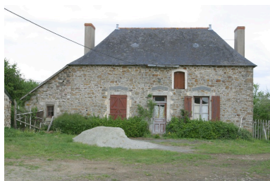
Le logis. Phot. François Lasa IVR52_20035301495NUCA
