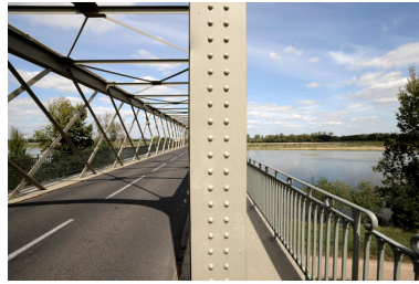
Rivets Phot. Bruno Rousseau IVR52_20114902453NUCA
