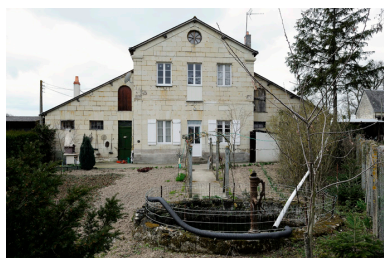
Façade principale Phot. Bruno Rousseau, Phot. Youenn Communeau IVR52_20114900697NUCA
