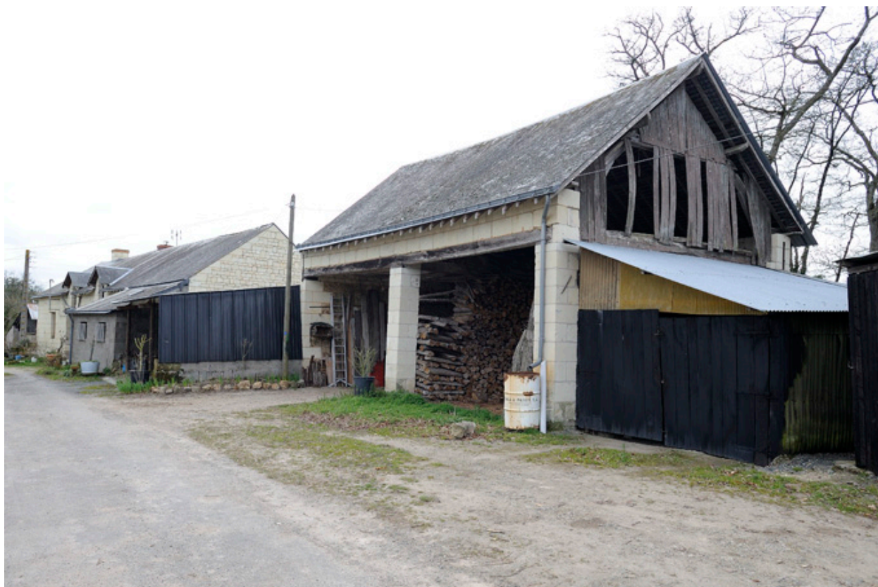
Grange, remise, communs
