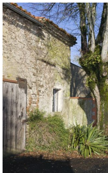
Le pigeonnier : facade est. 17e-18e siècles. Phot. Yves Guillotin IVR52_20104403047NUCA
