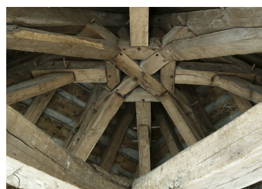
Charpente du pigeonnier. Phot. Patrice Giraud IVR52_20088500932NUCA
