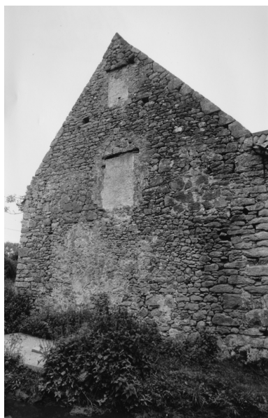
Logis nord. Pignon ouest, 1990. Phot. Denis (reproduction) Pillet IVR52_20094401382NUC
