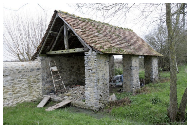
La seconde remise. Phot. François Lasa IVR52_20075301331NUCA
