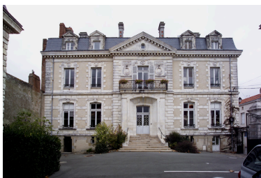
La façade sud. Phot. Denis Pillet IVR52_20034401921NUCA
