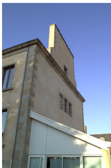
Pignon occidental. Phot. Denis Pillet IVR52_20054402260NUCA
