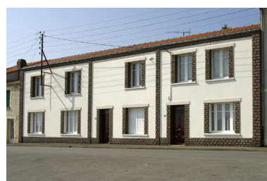
14, 14 bis quai Edmond-Libert. Phot. Denis Pillet IVR52_20034400245NUCA
