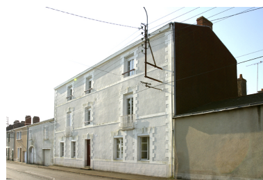
49, quai Chassagne. Phot. Denis Pillet IVR52_20034400192NUCA
