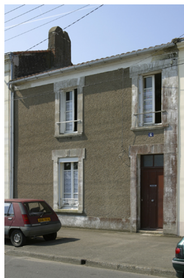
6, quai Edmond-Libert. Phot. Denis Pillet IVR52_20034400254NUCA
