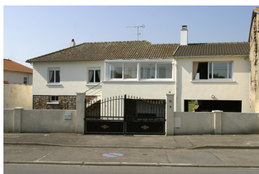
19, quai Chassagne. Phot. Denis Pillet IVR52_20034400233NUCA
