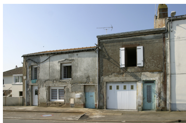
20, 21, quai Chassagne. Phot. Denis Pillet IVR52_20034400232NUCA
