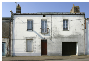
22, quai Chassagne. Phot. Denis Pillet IVR52_20034400231NUCA
