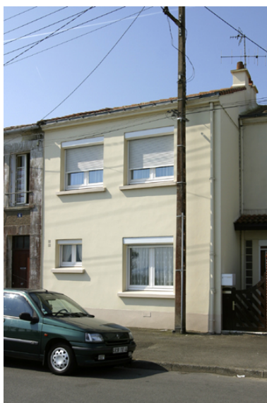
6, quai Edmond-Libert. Phot. Denis Pillet IVR52_20034400253NUCA
