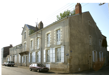
51, quai Chassagne. Phot. Denis Pillet IVR52_20034400189NUCA
