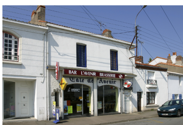
9, quai Edmond-Libert. Phot. Denis Pillet IVR52_20034400251NUCA
