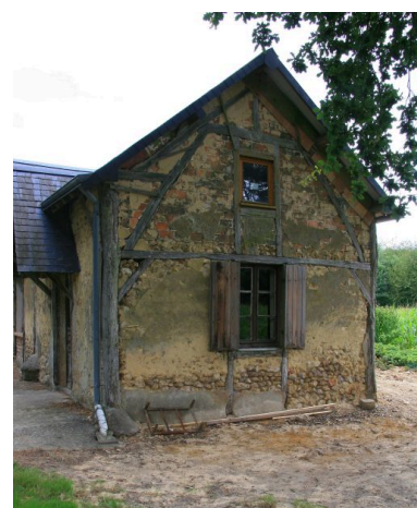
Pignon. Phot. Jean-Baptiste Darrasse IVR52_20087202004NUCA
